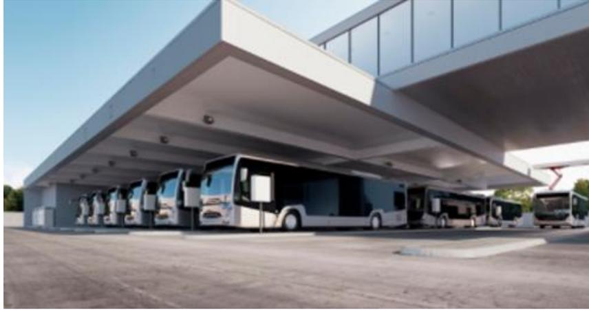
Another possible design would be overhead plug-in charging. In this design, the buses are parked in lanes and a structure is built over the parking lanes, similar to the example shown in **Figure 1-3**.
